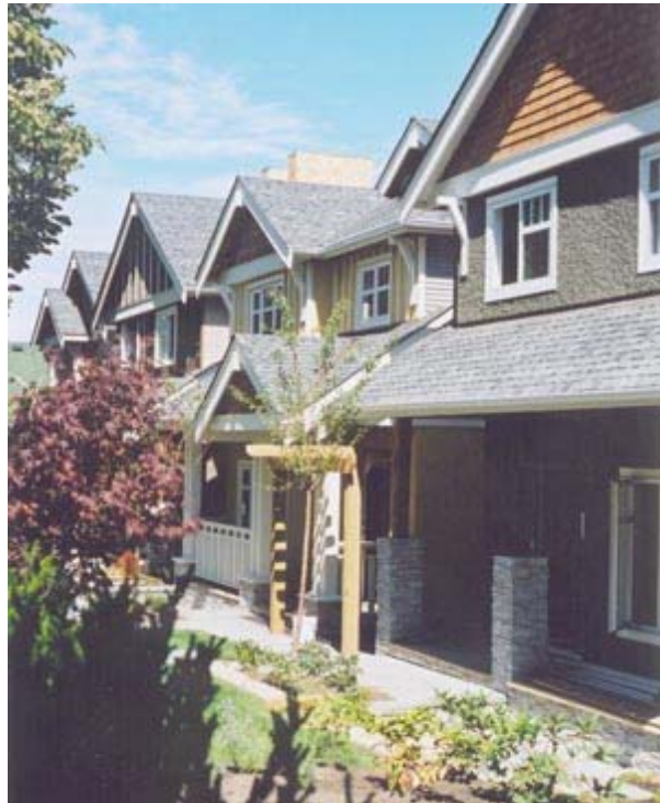
BRITCO STRUCTURES built the 20 modules for the 5 home infill project at Riley Park in the City of Vancouver
